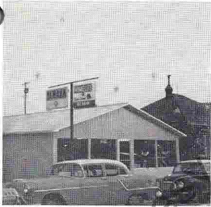
Exterior of new shop "The Basin"
