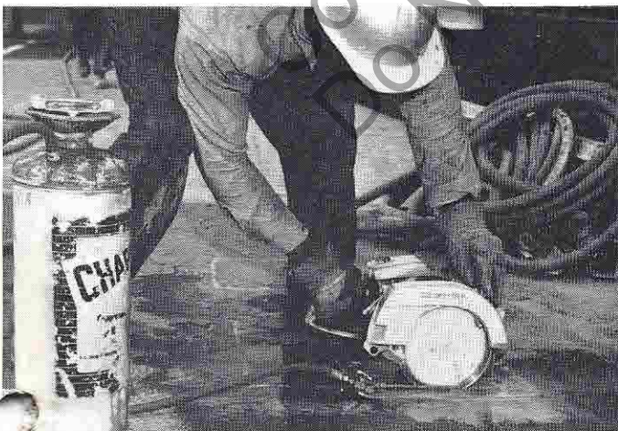
An XL-100 circular saw with Diamond Blade and water attachment is being used here to score a section of pavement which is to be removed.
