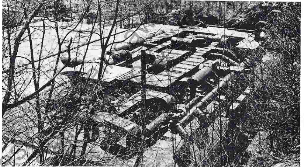
View of the roof of the new Test Lab in Port Chester, shows the maze of ducts, pipes and smoke stacks which are necessary for a safe, efficient operation.
