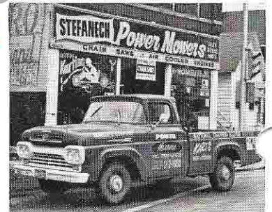
Exterior of Stefanech Mower Service, with service truck.
