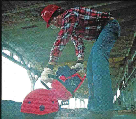
Cuts openings in prestressed textured concrete panels.
