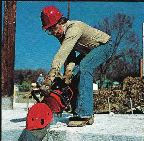
Cuts expansion joints in curbs and sidewalks.
