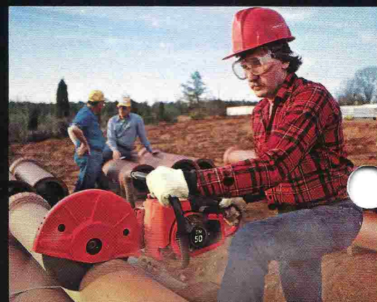
Makes a clean cut in drainage tile.
