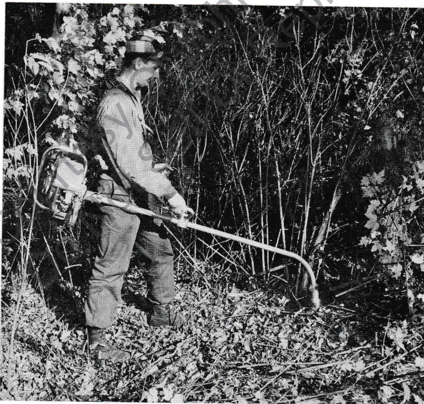
Figure 10—Brush Cutter In Action
