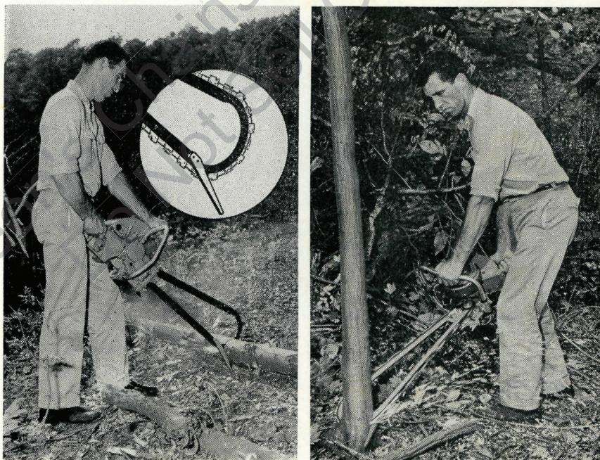
Figure 9—Bucking and Felling With Clearing Attachment
